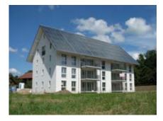
Figure 19: 100% solar heated multi-family house in Switzerland. Installed capacity 193  $kW_{\rm fh}$  (276 m<sup>2</sup> collector area) and a 205 m<sup>3</sup> heat storage. (Source: Jenni Energietechnik AG, Switzerland)
