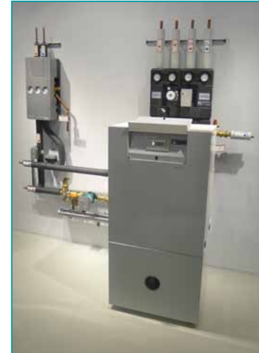
Figure 37 - Central element of an hybrid system combining geothermal and solar thermal technology (© EHPA)
