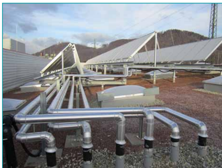
Figure 40 - Large-scale hybrid system combining solar thermal and heat pump technology to provide space heating with high solar fraction to a commercial building (© Austrian Institute of Technology).
