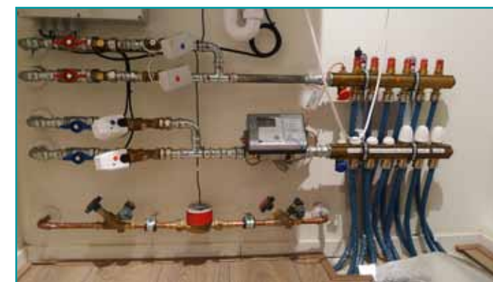
Figure 20 - integrated control of the heating system (© Thomas Nowak, EHPA)
